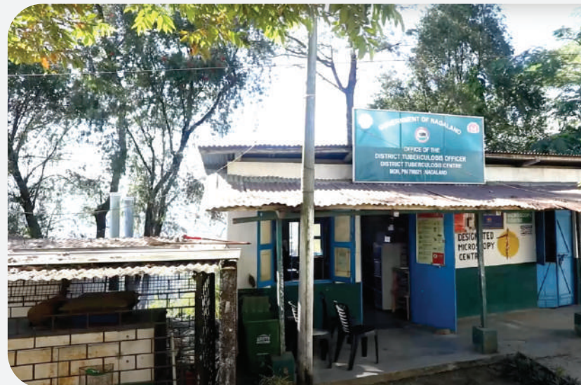
The office of the District TB Officer in Mon, Nagaland, also serves as a clinic for TB patients. The clinic, which doubles as an office, is located separately, opposite the main hospital building.
